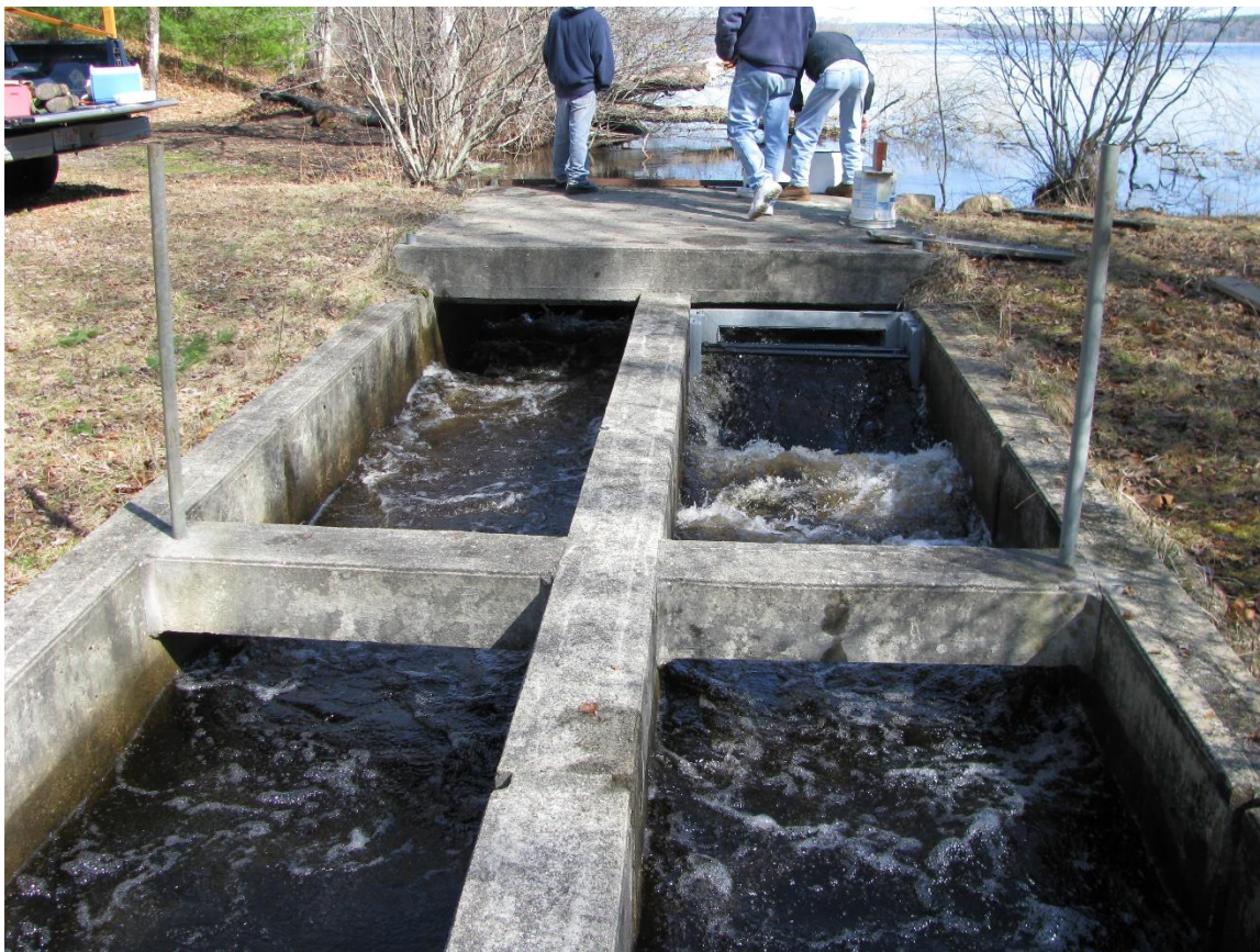
Ladder at the outlet of Snipatuit Pond
